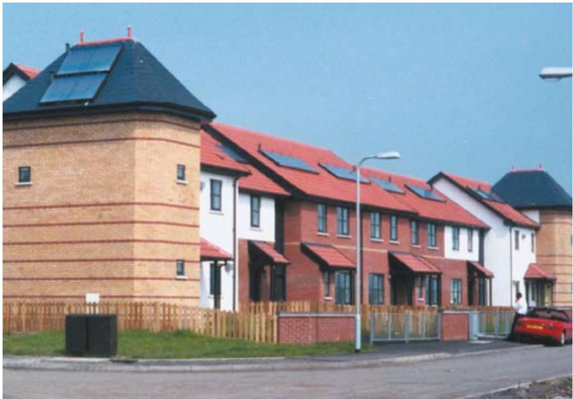
Figure 1 Roof-mounted collectors on Gorseinon development
