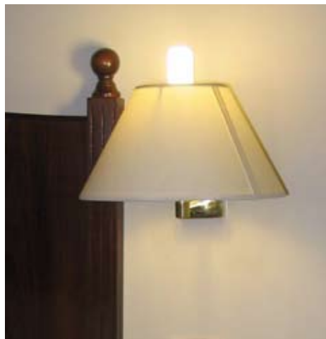
Figure 5 Example of poorly matched lamp and luminaire. The lamp was also 3500K – far too cool for a hotel bedroom
