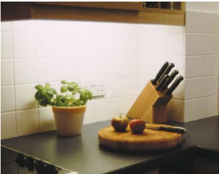
Figure 8 Under-cabinet lighting improves safety on work surfaces as well as having a high degree of permanence
