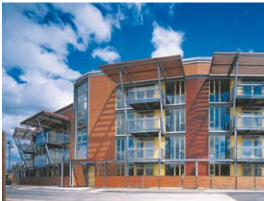
An example of permanent shading to reduce solar gains. Greenwich Millennium Village Phase 2a, Proctor & Matthew (photo: David Churchill)
