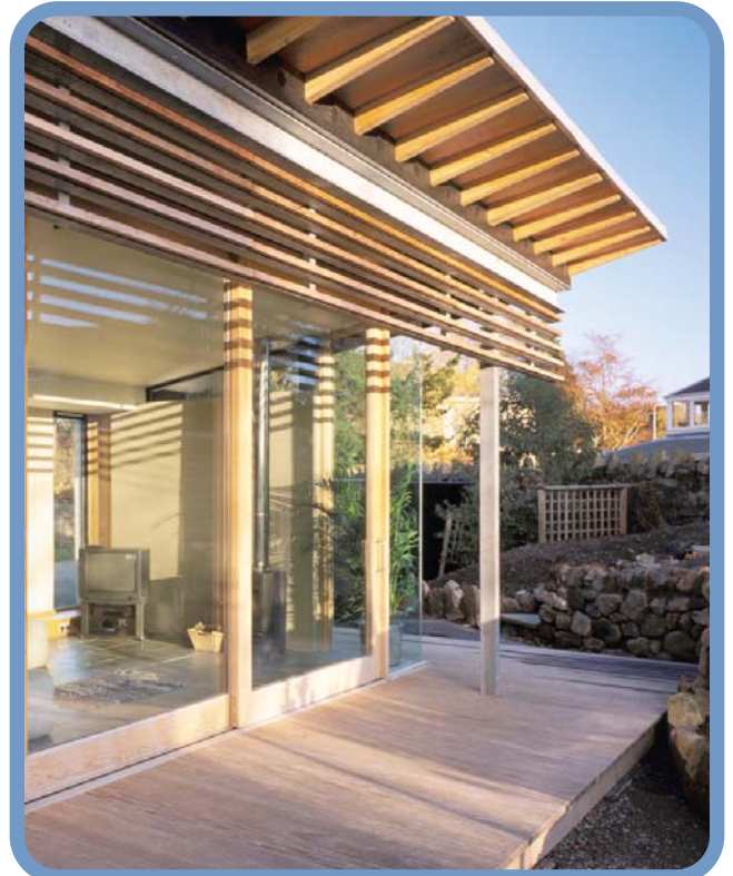
Rising overhang and horizontal louvres combine to shade summer sun. House extension, Reid Architecture. Photo: Andrew Lee Photography
