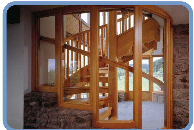
A stone wall and slate floor providing mass in a timber frame house - Dragon house, Herefordshire, Constructive Individuals. Photo: Philip Bier
