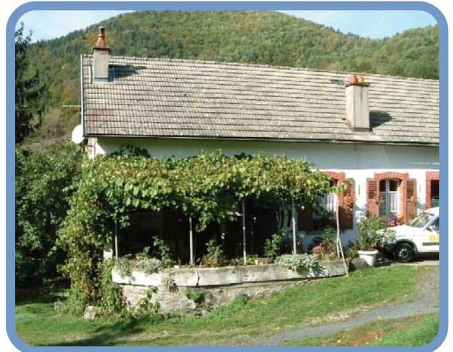
Vegetation needs to be maintained if it is to be used for shading! Photo: John Willoughby
