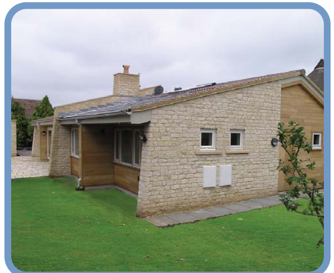
Setting back the façade allows different degrees of shading to be provided. Low energy bungalow, Cheltenham, Buchanan Partnership. Photo: Bruce Buchanan
