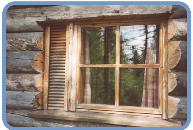
Side vents to windows can provide secure night ventilation. Log cabin, Finland. Photo: John Willoughby
