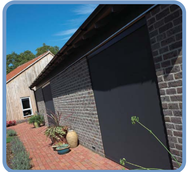
External roller blinds can be discreetly accommodated in the dwelling structure. Lynn Road, Mole Architects. Photo: Reeve Photography
