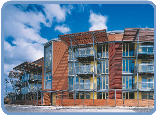
Permanent shading such as louvres work particularly well in urban settings. Greenwich Millennium Village Phase 2a, Proctor and Matthew. Photo: David Churchill
