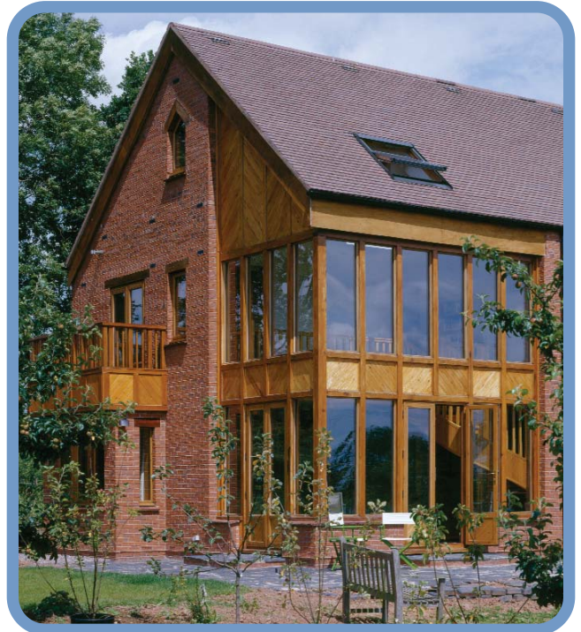
Rooflights are a useful way of providing night ventilation. Dragon house, Constructive Individuals. Photo: Philip Bier
