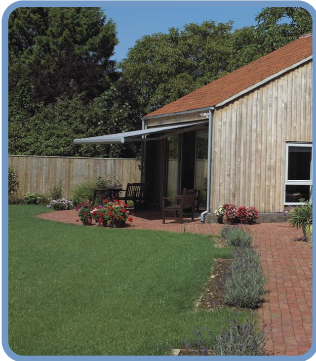
Awnings can be highly effective and allow continued access to the building. Lynn Road, Mole Architects. Photo: Reeve Photography
