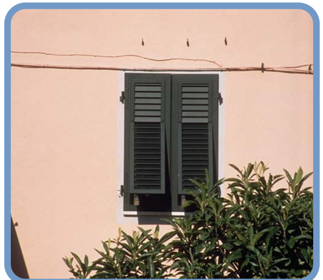
Traditional shutters, or persiane, are common abroad and provide shading and ventilation. Photo: ATLL, www.atll.it
